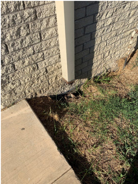
Downspout Rusted
