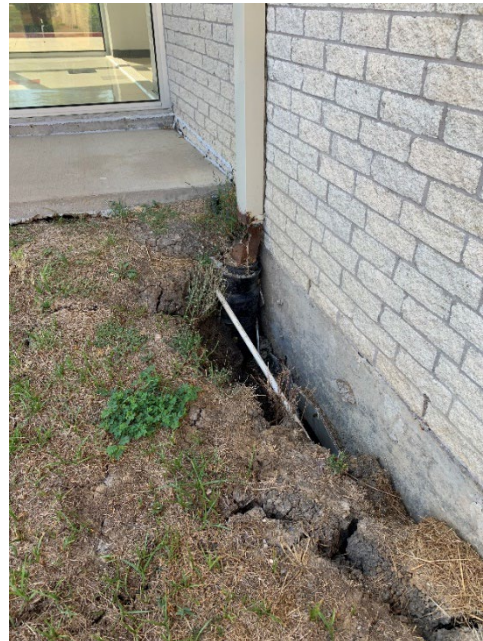
Erosion at Sidewalk and Foundation
