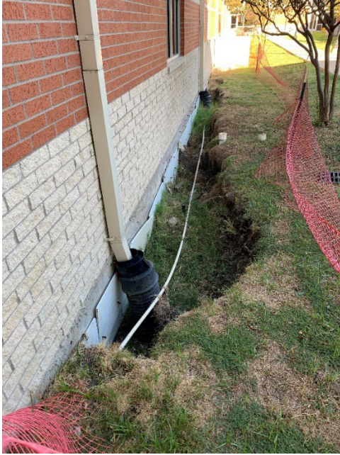
Erosion at Perimeter Grade Beam
